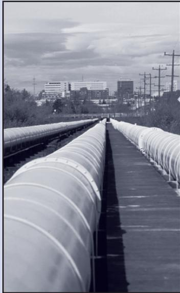
Four large transmission lines carry the water from Chaplain Reservoir to Everett. Each pipe is four feet in diameter and can carry about 50 million gallons of water a day. Three lines
