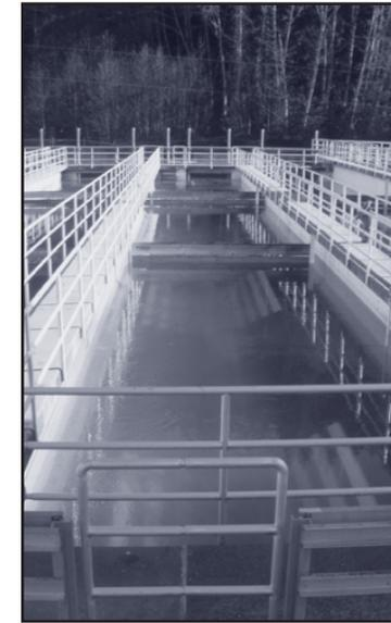
From the late 1920s through the early 1980s, the drinking water from Chaplain Reservoir was treated by screening and chlorination. In 1983, a \$30 million Water Treatment Plant was built on the south end of Chaplain Reservoir. This state-of-the-art plant uses advanced filtration processes to remove possible contaminants and chlorination to make
