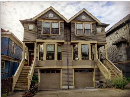
Figure 9-5: The main entrance is more than 4 feet above average grade
