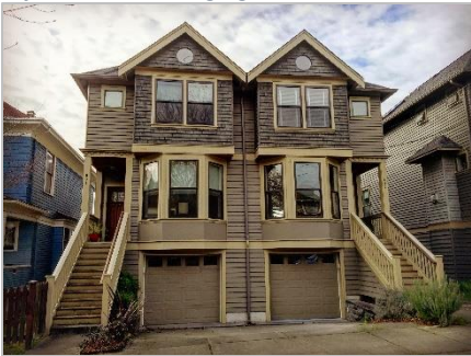
Figure 9-6: The main entrance is more than 4 feet above average grade
